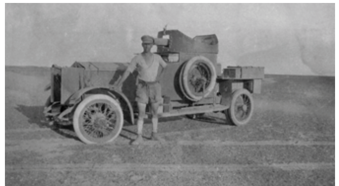
A Rolls-Royce armoured car with half the revolving turret removed in order to improve ventilation in the desert conditions.
