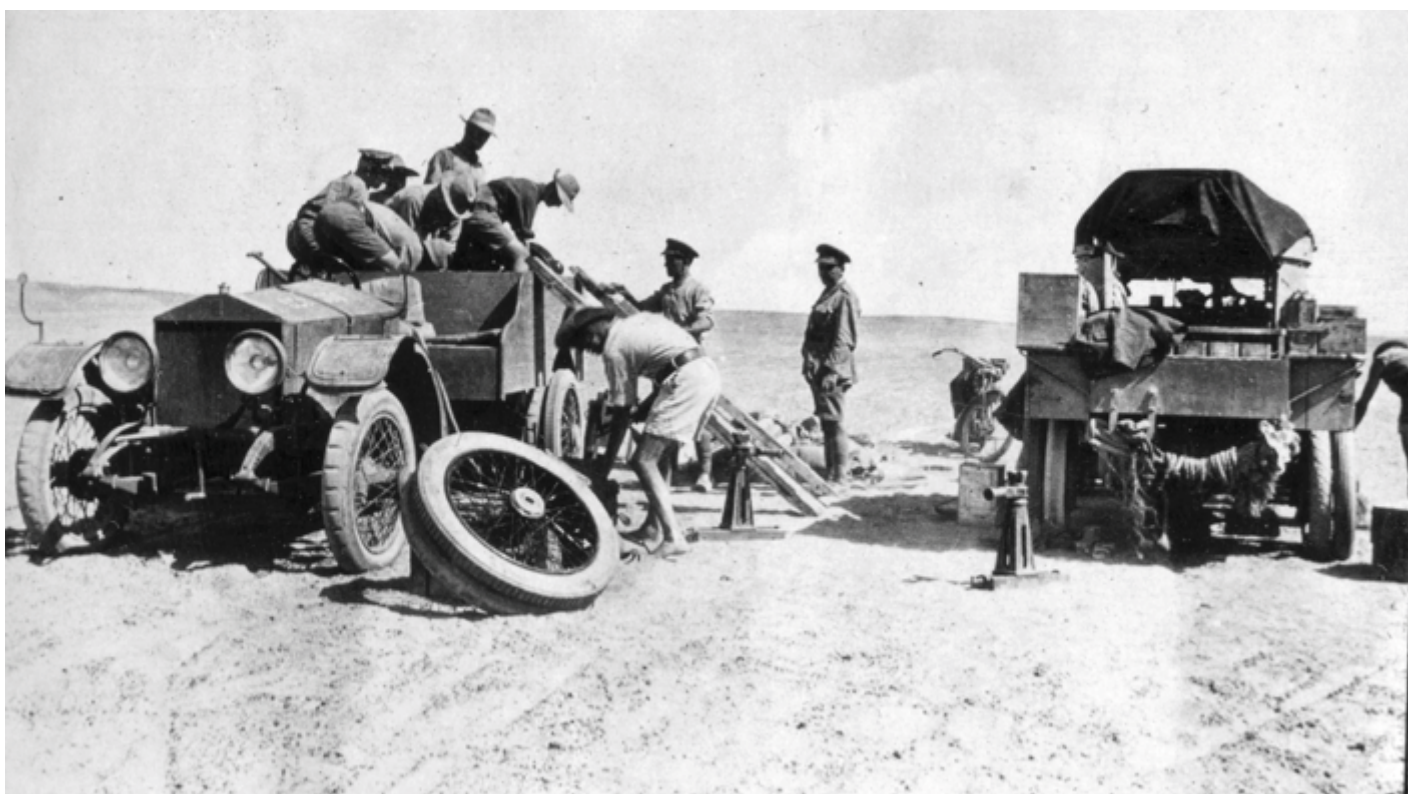
Desert repairs required of a box-bodied Rolls-Royce. At a minimum, the vehicles always travelled in pairs.
