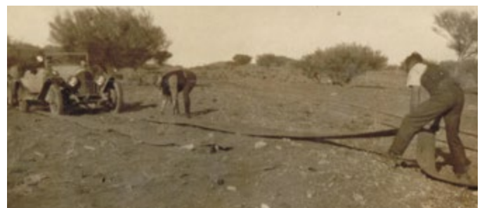
Adjusting matting across the sandy ground towards railway lines at Lake Sand Hills on the Oodnadatta trip.
