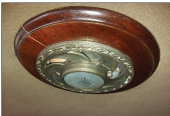
The interior light doubles as a vent for cigar smoke. Note the wasp nest lurking in there.
