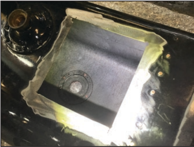
The inside of the tank required considerable cleaning. Following this the tank was patch repaired, refinished and painted before the inside was protective coated.
