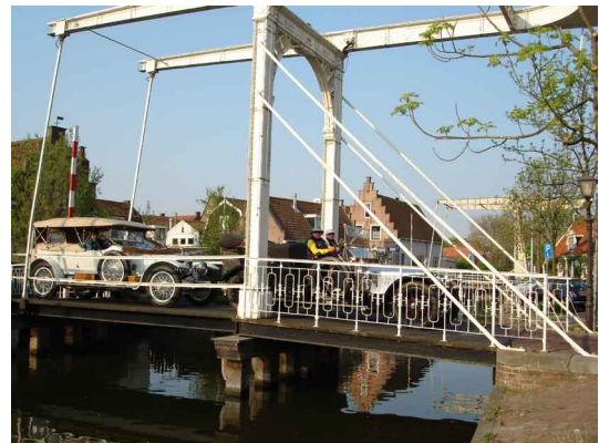
Hopefully the bridge will support the combined weight of cars
