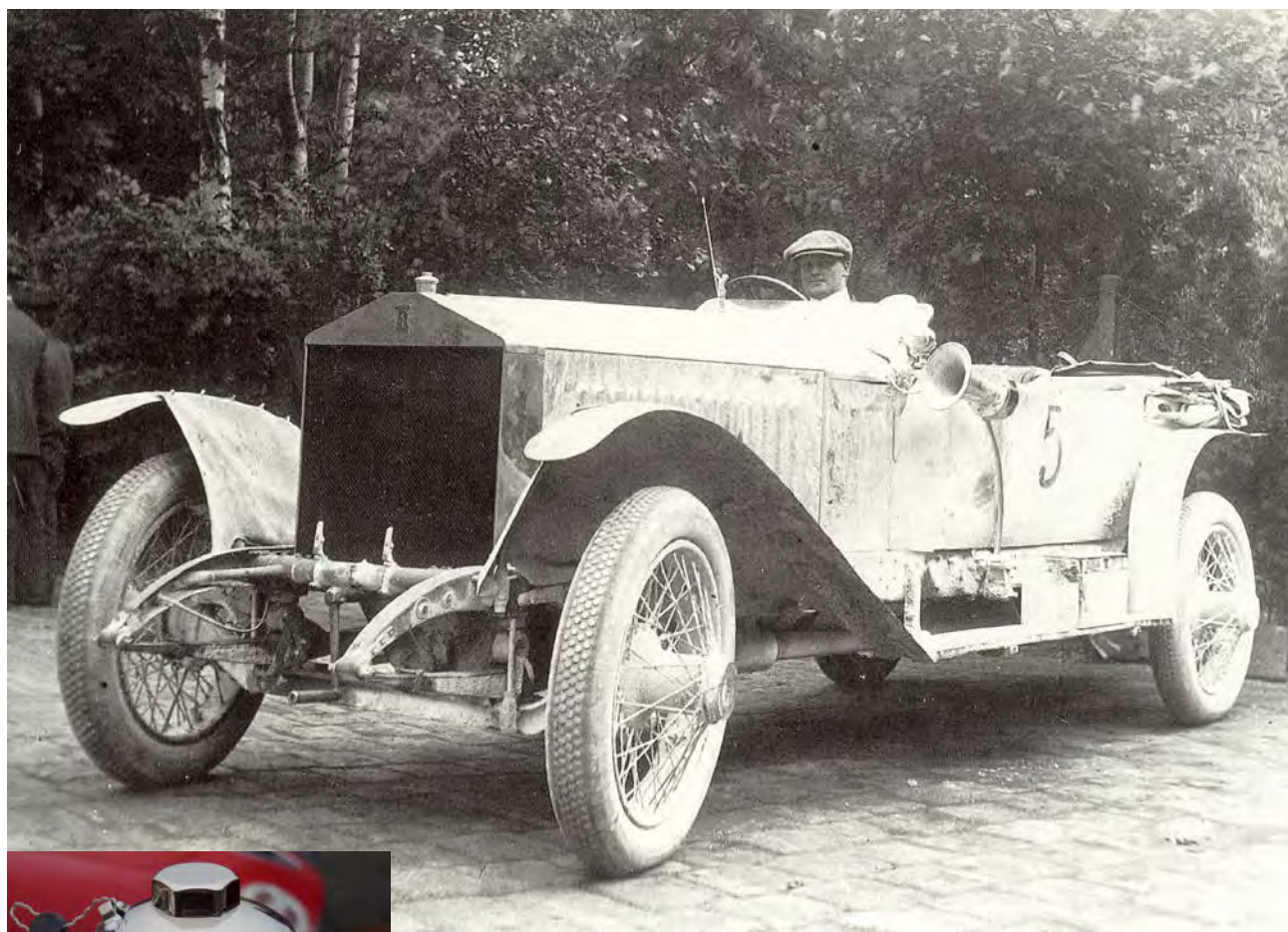
Rolls-Royce test department's H.A. 'Tubby' Ward on 18PB - the body, by Radley's own company Portholme was designed for lightness with no doors and no under-chassis braces, lightweight mudguards with canvas valances to protect the driver from mud and stones and rubber bump protectors over the front springs.
