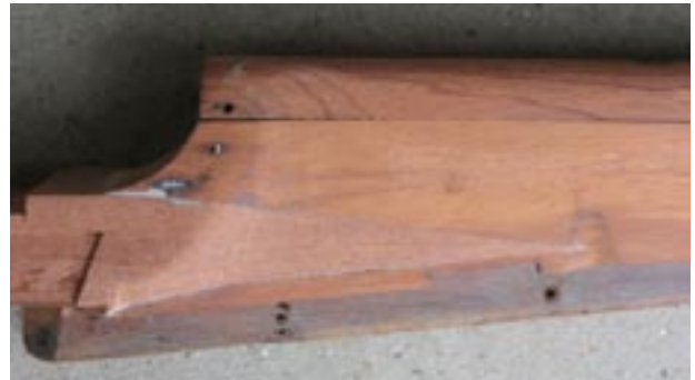
new piece spliced into original front A-post
