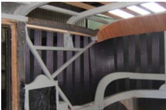
structure repaired & primed
