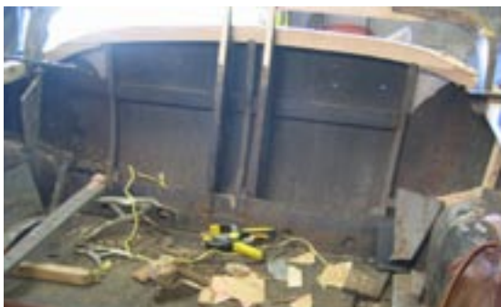
back being repaired
