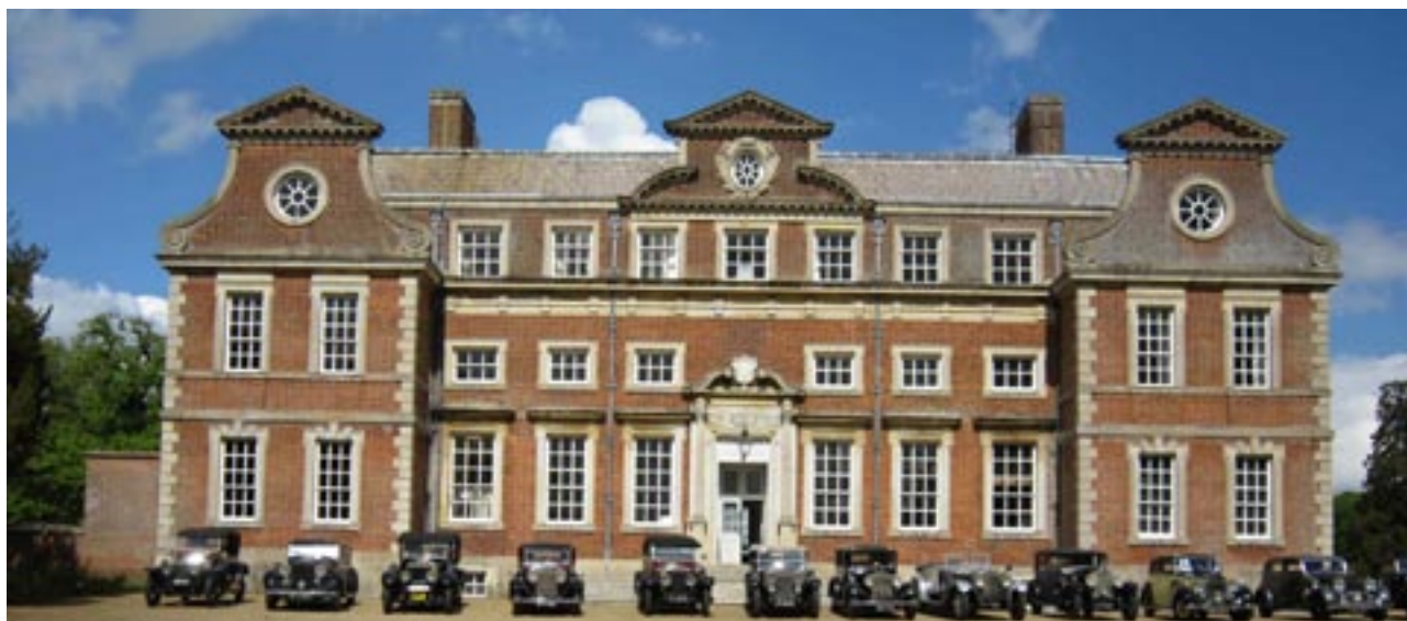
The cars in front of Raynham Hall, seat of the Marquesses Townshend
