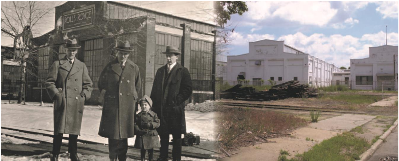
The Rolls-Royce plant at Springfield Massachusetts... then and prior to demolition in 2011
