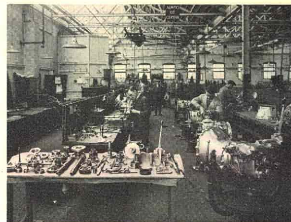
Gear box erection bay. Note hanging slogan, one of many throughout the works
