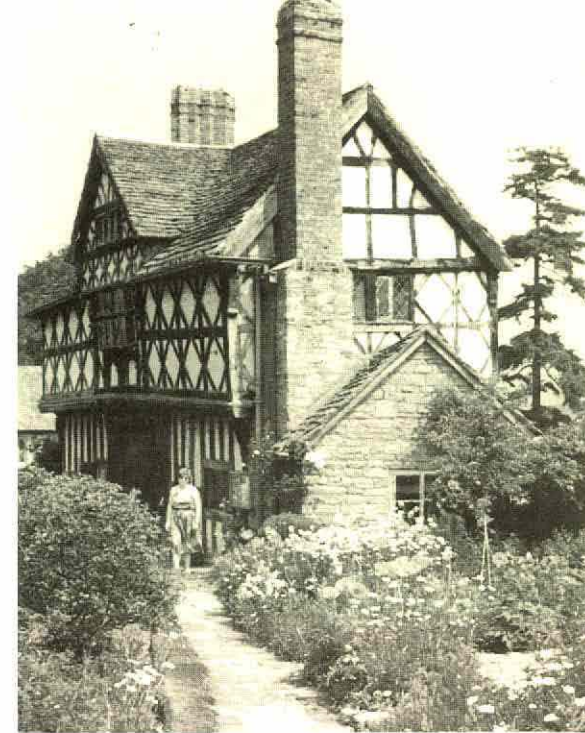
Gatehouse at Stokesay Castle Photograph John Kennedy
