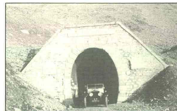
1922 Ghost at Parpaillon tunnel in 1989 Photograph by John L. Kennedy
