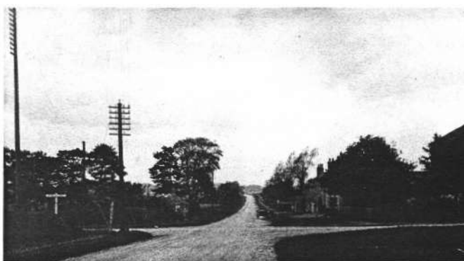
The Bramham Moor crossroads on the Great North Road, seen on 17 May 1912, a rather fine surface for easy motoring in 1701. These superb late 18th century roads had been surfaced with a finely ground granite resulting in the white appearance. Horses and wagons did no damage but motor tyres and speeds eventually degraded the surfaces. (Courtesy of Leeds City Council photographic archives)
