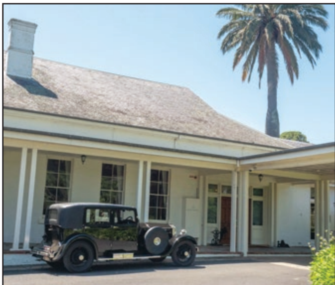
Noel Baker 20hp, GTM10 in front of Chateau Yering. The palm tree behind the house was planted in 1867 and is listed in the Register of Significant Trees in Victoria. Both the house and the gardens are listed for protection by Heritage Victoria.
