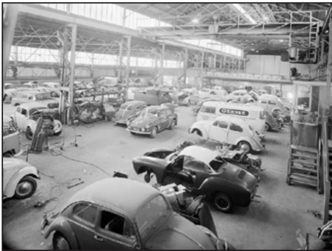
The VW plant at Clayton in 1969 which first produced Volkswagen Beetles in 1954. It was demolished recently to make way for a data centre. (Photo: Monash Public Library)
