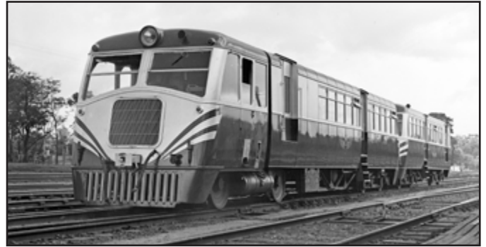
A Walker railcar. Walker railcars were of 153hp and were a combination of power units built by the Walker Railcar company, Wigan England and bodies built Martin & King. Pictured in Woodend 1948. (Photo: SLV)
